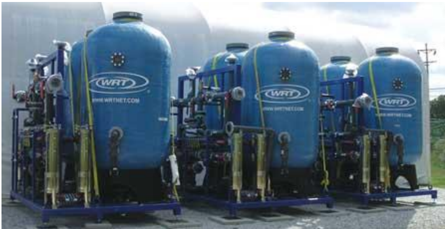
Radium-contaminated water is treated by passing through a fluidized ion-exchange bed of zeolite-based treatment media, a natural industrial mineral substance onto which the radium attaches.
