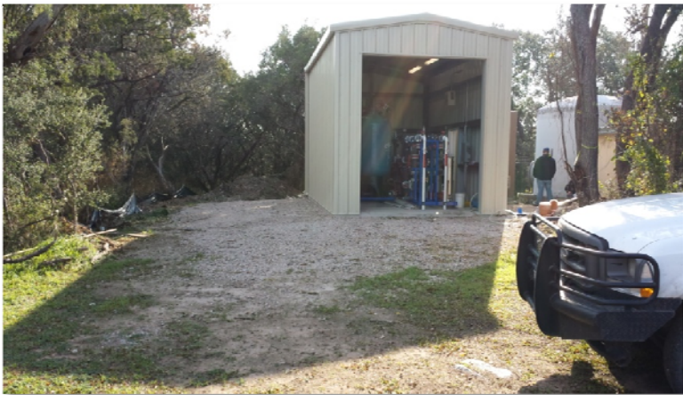
Tow Village radium removal system treatment building
