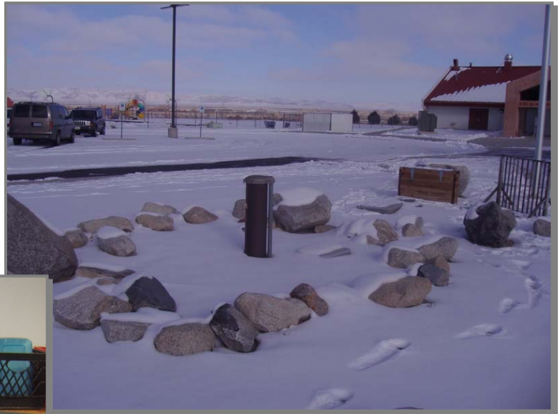
Schurz Elementary School's Z-92 ® /Z-33 ™ treatment system.
