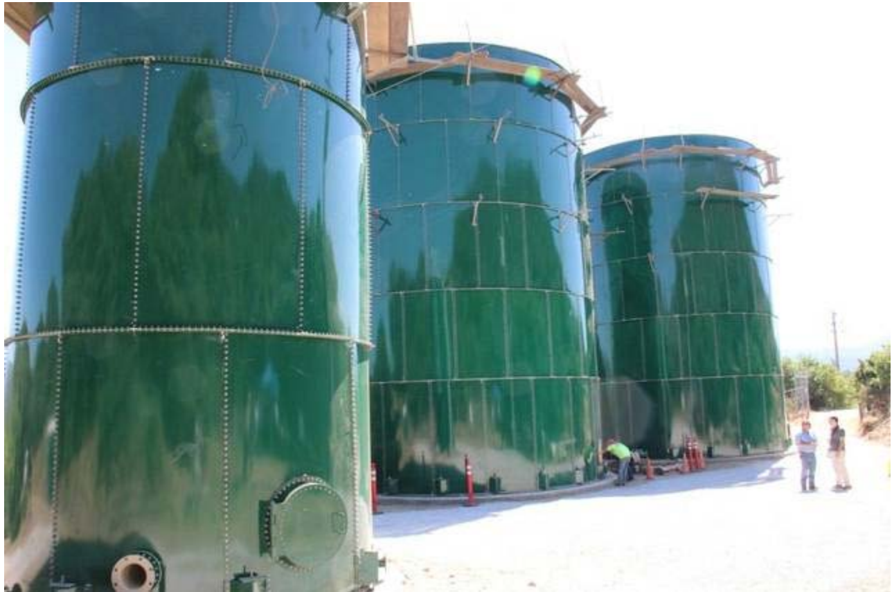
These three new water tanks are part of the $20 million upgrade taking place with Hillview Water Company. The tank on the left is a 21,000 gallon backwash tank and the other two are 220,000 gallon storage tanks that are about six stories tall. The tanks are located at the soon-to-be-built water treatment plant off Victoria Lane. (Brian Wilkinson Sierra Star)
