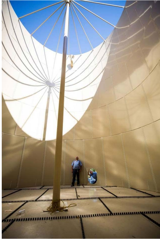
Two Hillview Water Company employees check out the inside of one of the new water storage tanks that will hold 220,000 gallons when filled. (Michael Costa Special to Sierra Star)
