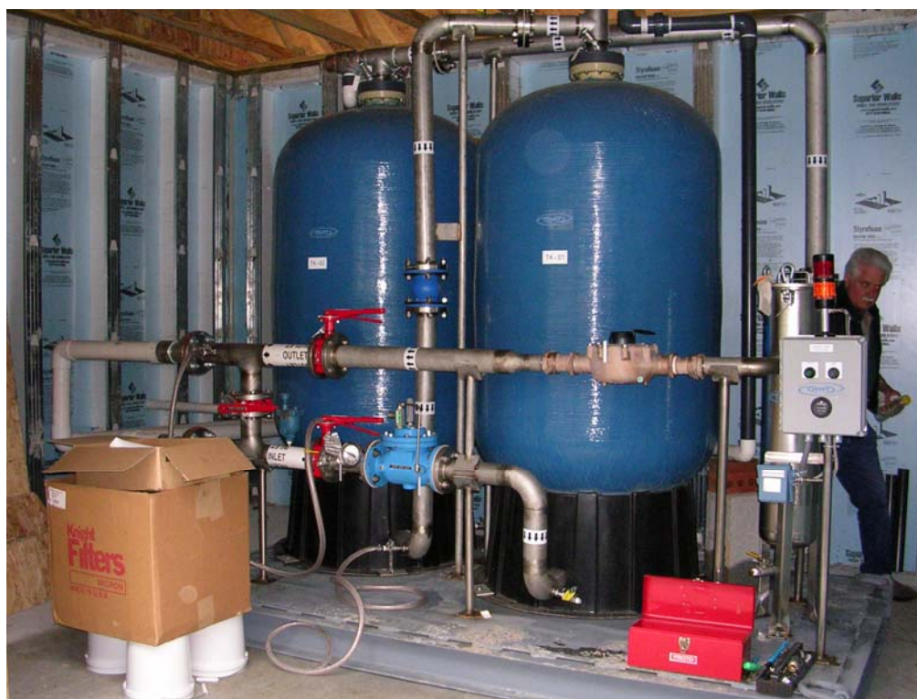
Figure 1 – Uranium removal units at Chesdin Manor
